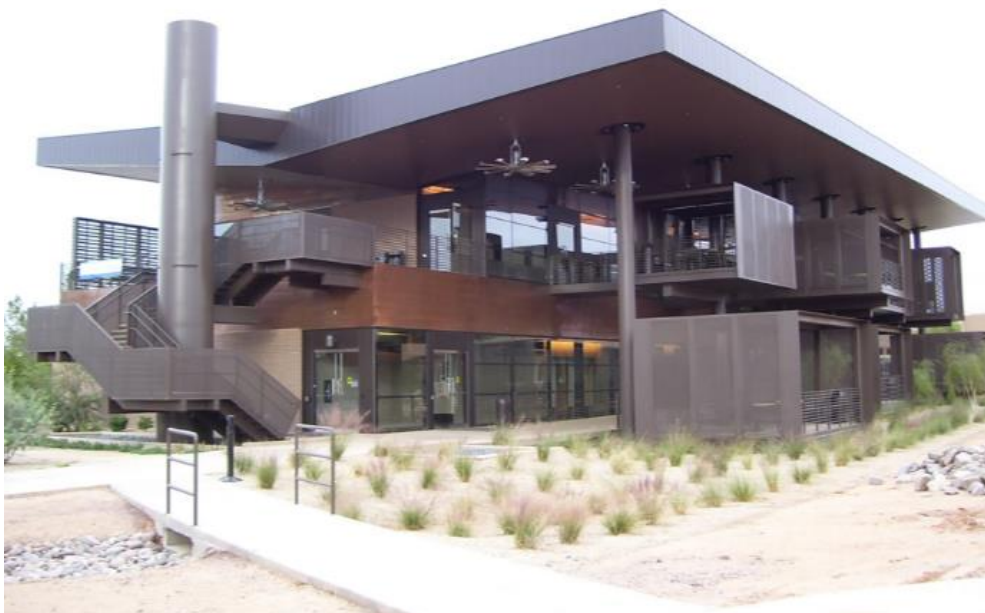
Paradise Valley Community College Life Science Building
